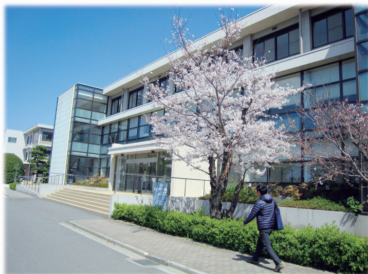
The Faculty of Integrated Arts and Sciences Building No.1
